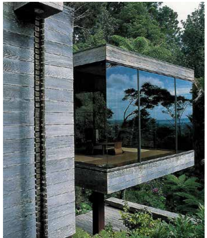
A large, glass-sided, tatami-matted room projects out into the bush and contrasts with the home's cedar exterior, chosen to weather in time and attract moss.
