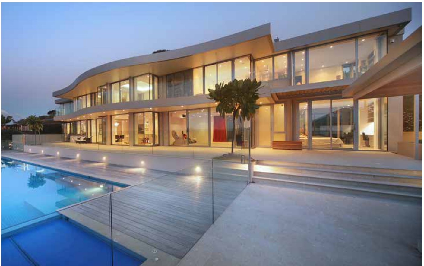
Farm Cove's living room, kitchen, theatre, and guest bedroom open to a large tiled outdoor terrace and infinity pool. The pool and hot water are on an energy-saving, passive-heating system.
