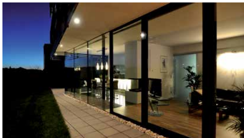
Triple-glazed, glass-only façades and a well-insulated wood structure minimize heating costs.
