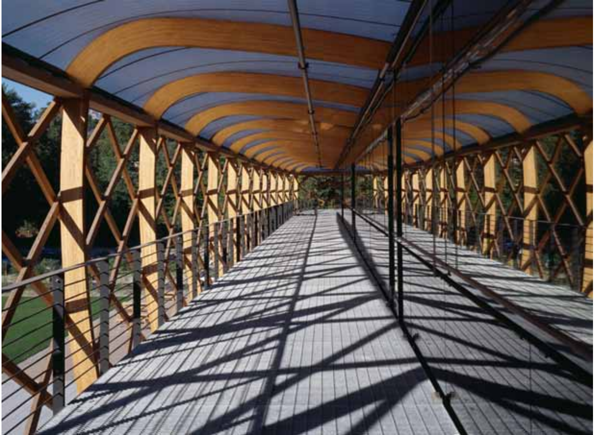
Affixed to the balconies, diamond-latticed wood shields the building from sun and weather.
